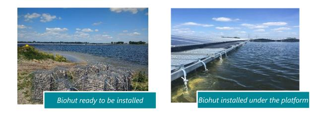
Since their installation, all modules remain well in place, without any visible impact on the floating structure or on its buoyancy. The Biohut do not show any sign of corrosion, and the substrate is well in place, with the presence of sediment inside the shell. The fouling of the mesh is low, so the modules did not need to be cleaned to keep the targeted ecological functions.
