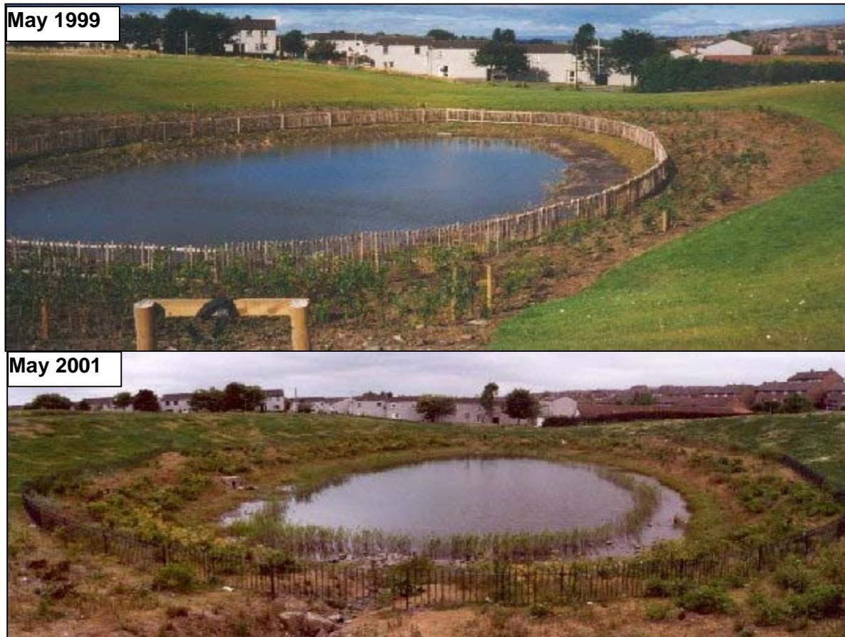
**Figure 4.3 Pond 6 – There are three ponds in a cascade**
