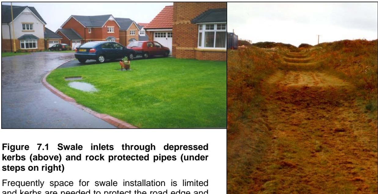
**Figure 7.1 Swale inlets through depressed kerbs (above) and rock protected pipes (under steps on right)**
