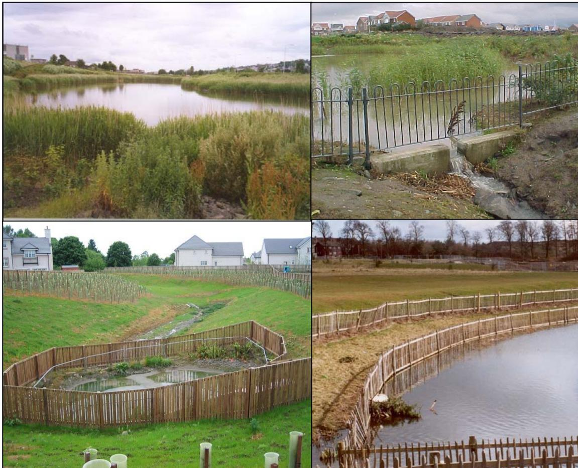
**Figure 5.4 Planted and erected barriers at three ponds and one detention basin (bottom left).**
