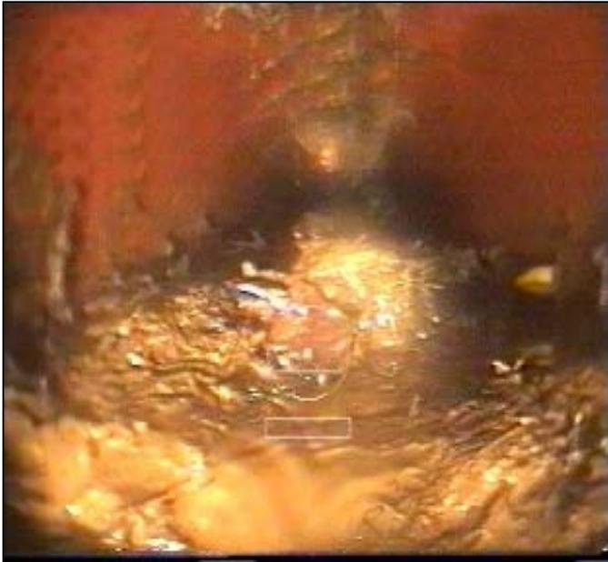
**Figure 8.7: Blocked Perforated pipe at Inlet to Filter Drain/ Filter Bed**
