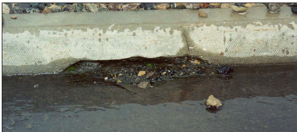
**Figure 8.11: Blocked Roadside Lateral Inlets**
