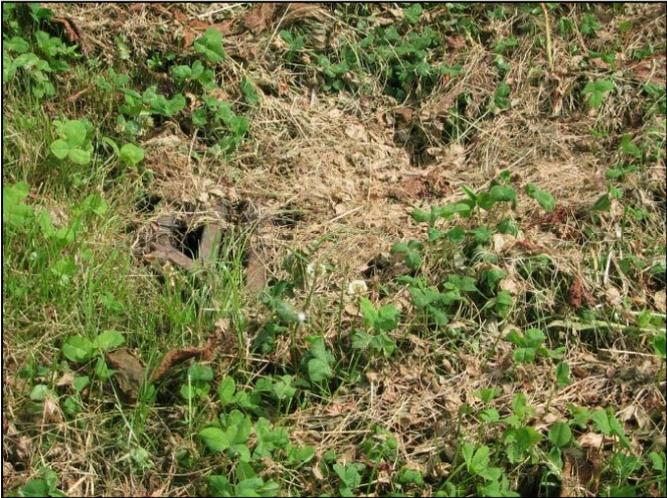
The fundamental principles of outlets are well known to design engineers. Unfortunately, several examples of blockage or potential blockage have been found and an example is shown in figure 6.2. It is apparent that insufficient thought is often given to access for blockage clearing. For example, manholes become surcharged making it impossible to clear a blockage. A further example is given in summary sheet 9.
