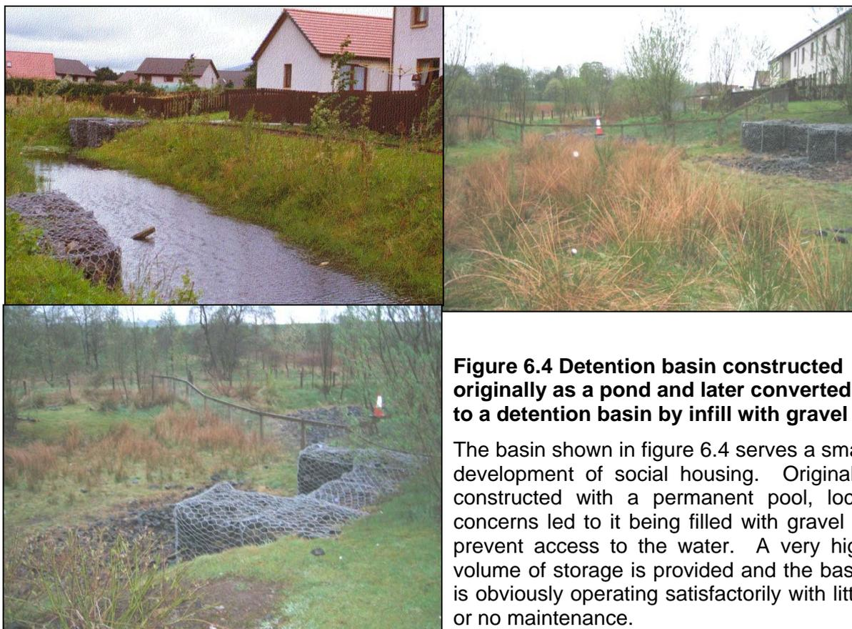
**Figure 6.4 Detention basin constructed originally as a pond and later converted to a detention basin by infill with gravel**
