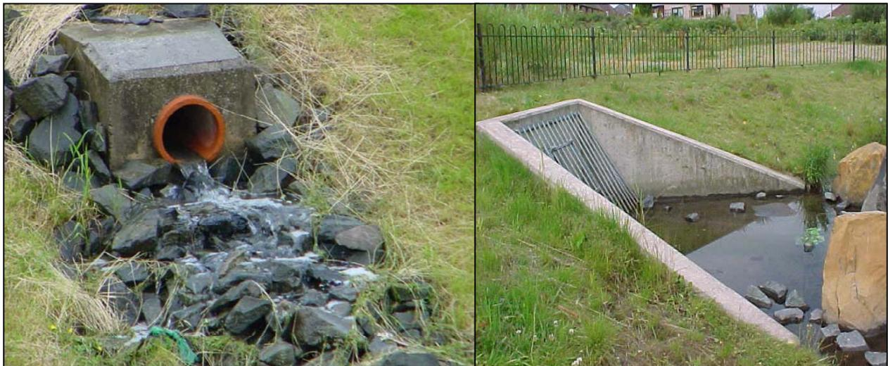
**Figure 5.1 Typical Pond Inlets** (equally applicable inlets are shown in figure 6.1)
