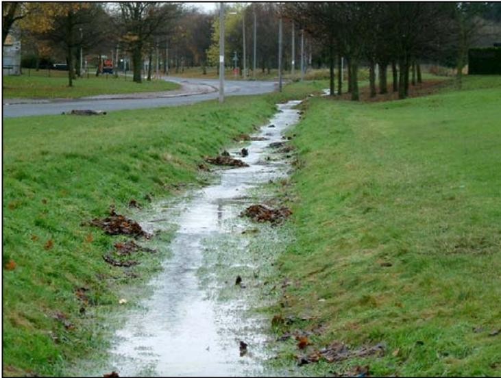
**Figure 4.21 Conveyance Swale in Ardler, Dundee**
