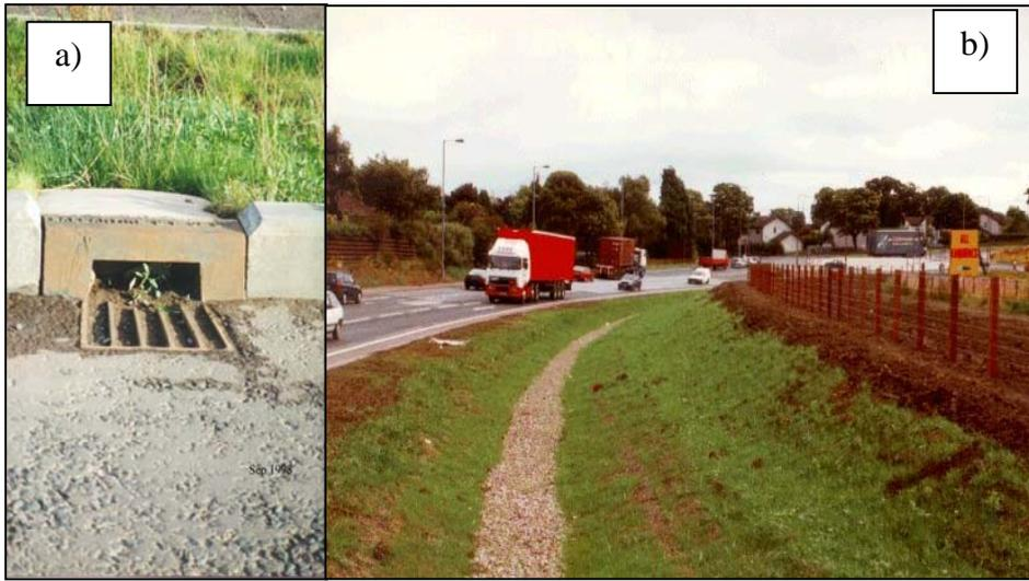
**Figure 7.2 Swale inlets** a) through Clearway units (no longer used due to frequent blockage); b) lateral inflow.
