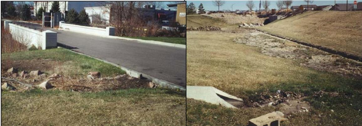
**Figure 12.1 Debris in runoff channel    Figure 12.2 Maintenance of detention basin base**
