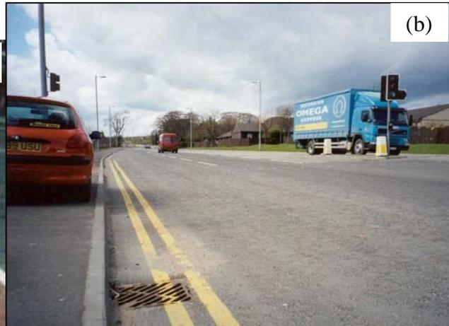
**Figure 8.1 Lang Stracht Filter Drain Site – 750m long draining all of the highway and parts of some side streets.**
