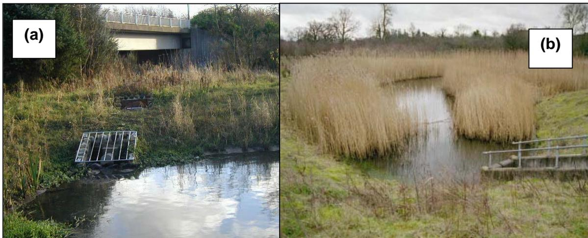
Figure 5.3 Exposed pond outlets using Hydrobrake (a) and Narrow vertical slot (b)
