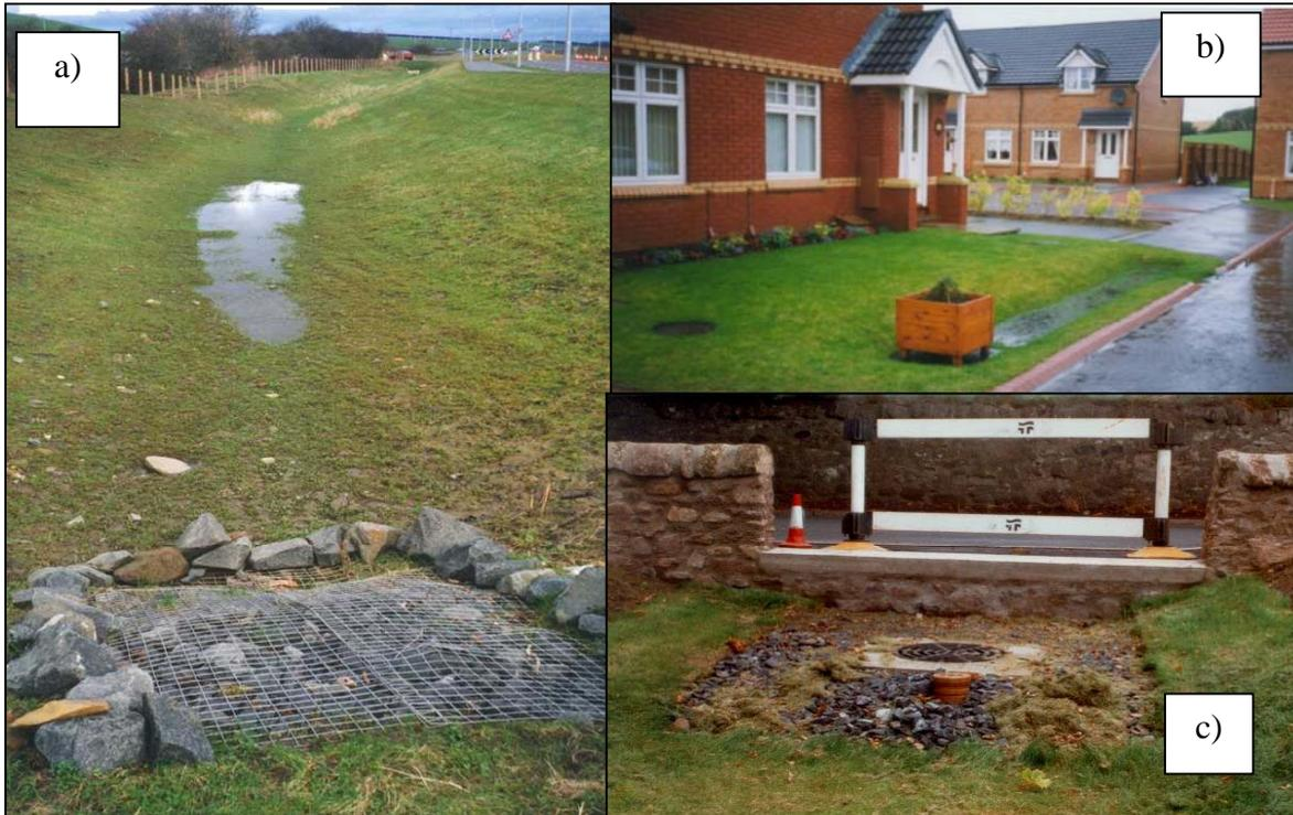
**Figure 7.3 Swale Outlet arrangements** a) small diameter pipe under rock protection in foreground; b) Planter placed to conceal grating on raised outlet to small roadside swale; c) Raised outlet at lower end of stepped swale illustrated in figure 7.1.
