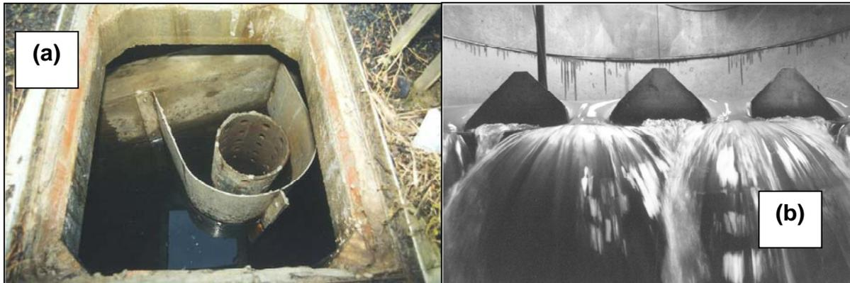
Figure 5.2 Underground pond outlets – (a) slotted standpipe pipe; (b) Multiple 90<sup>0</sup> Vee notches
