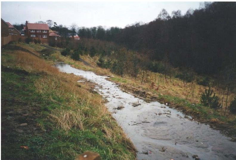
**Figure 12.6 Swale/ detention basin at Murieston, Livingston overwhelmed by construction stage runoff**
