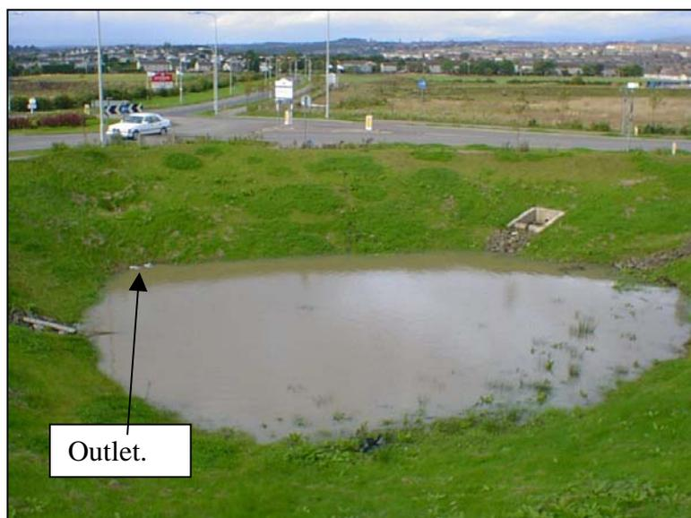
The outlet from this basin was blocked shortly after monitoring commenced. This was due to a large sheet of polythene becoming lodged at a location where access was not possible.
