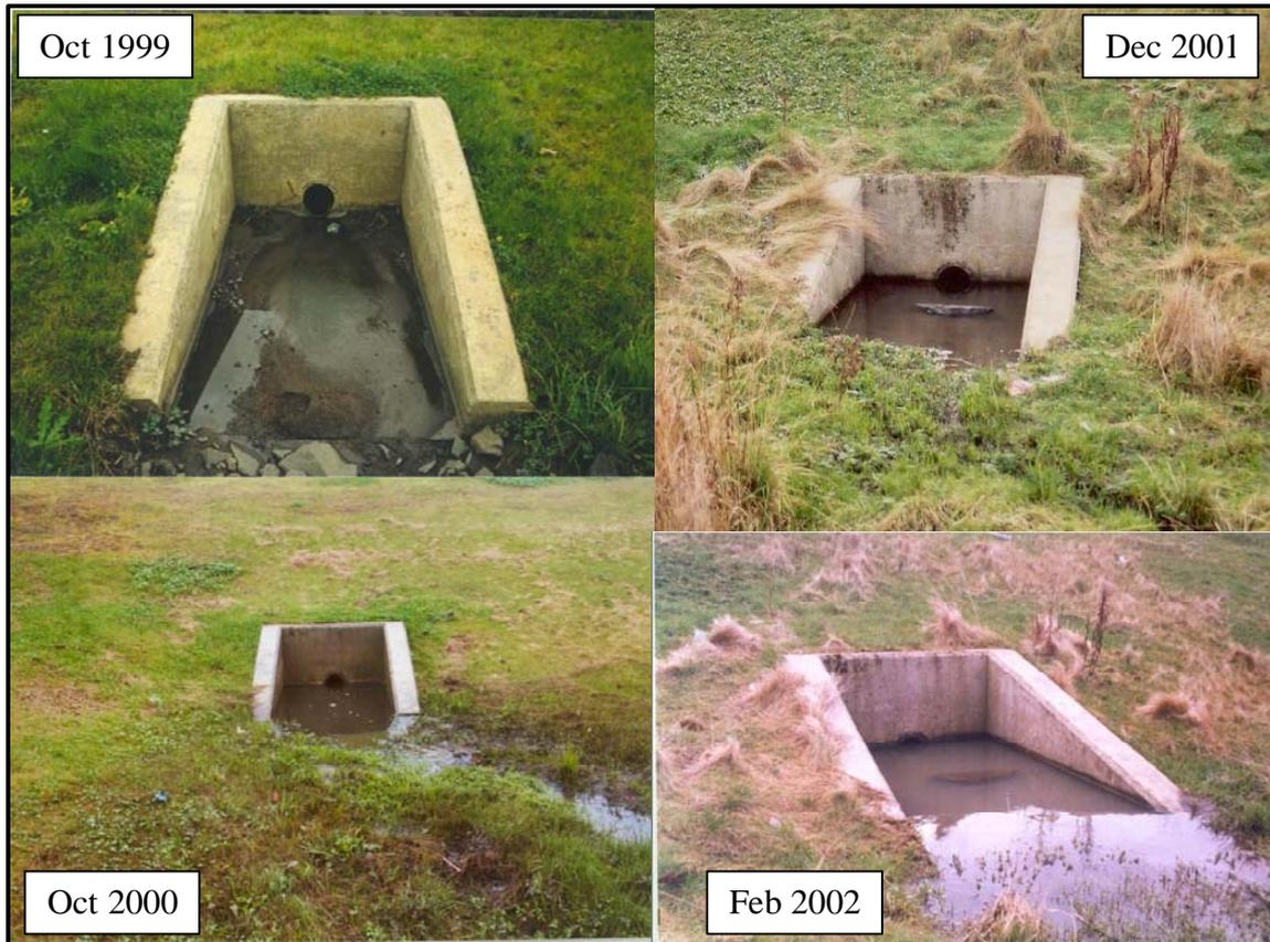
**Figure 8.4 Detention Basin D/M Sedimentation at Inlet**
