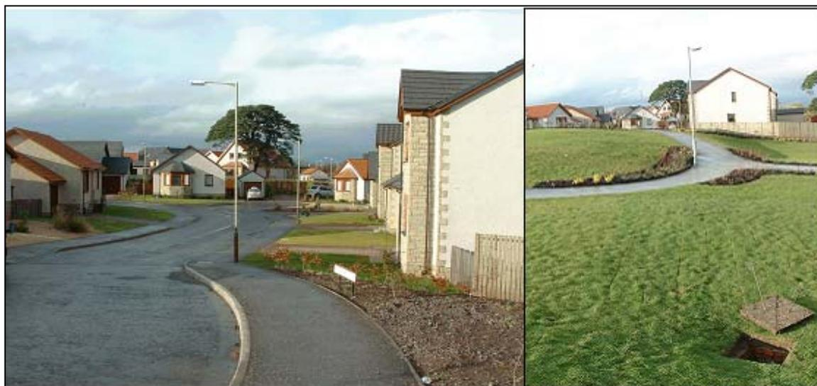
This filter drain is on a sloping site in primarily fill material. There is permanent water in the manholes due to the sealed manhole bases. The water table is below base of the system.
