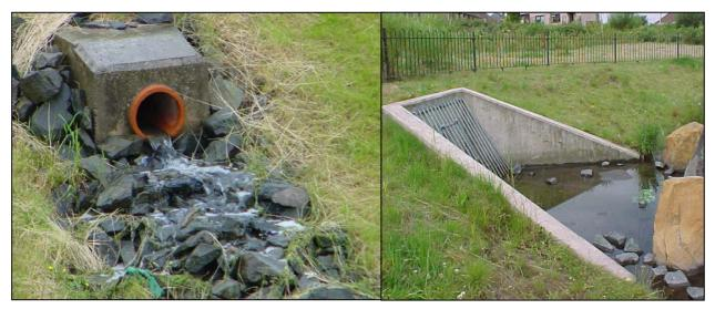
Figure 5.1 Typical Pond Inlets (equally applicable inlets are shown in figure 6.1)
