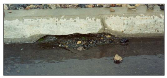
Figure 8.11: Blocked Roadside Lateral Inlets
