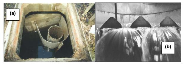
Figure 5.2 Underground pond outlets – (a) slotted standpipe pipe; (b) Multiple 90<sup>0</sup> Vee notches
