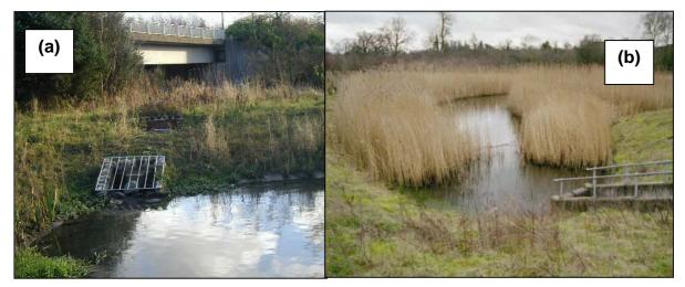
Figure 5.3 Exposed pond outlets using Hydrobrake (a) and Narrow vertical slot (b)
