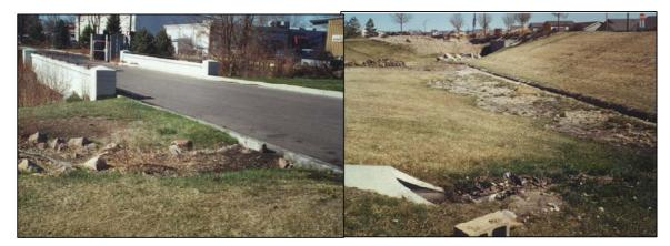
Figure 12.1 Debris in runoff channel Figure 12.2 Maintenance of detention basin base
