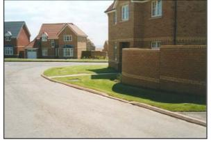
Roadside detention basins produce an undulating appearance to the road margins and are relatively easily maintained. Surveys have shown that there is little resistance from residents even though they are periodically full of water. Figure 4.19 shows two further examples.
