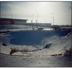
2001 leading to areas absent of vegetation, which was unsightly and can hardly be considered to be satisfactory. Erosion at one inlet became noticeable with a channel appearing to the side of the inlet. Sediment which is accumulating at the outlet is probably being scoured from the areas with no vegetation within the basin, from the gullying at an inlet and fine sediments from road runoff.
