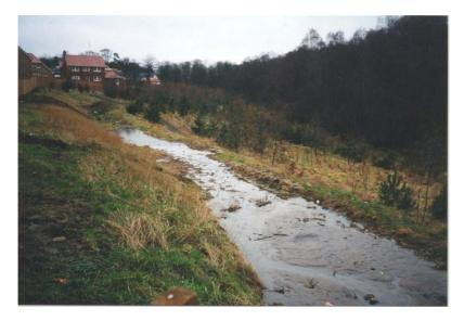
Figure 12.6 Swale/ detention basin at Murieston, Livingston overwhelmed by construction stage runoff
